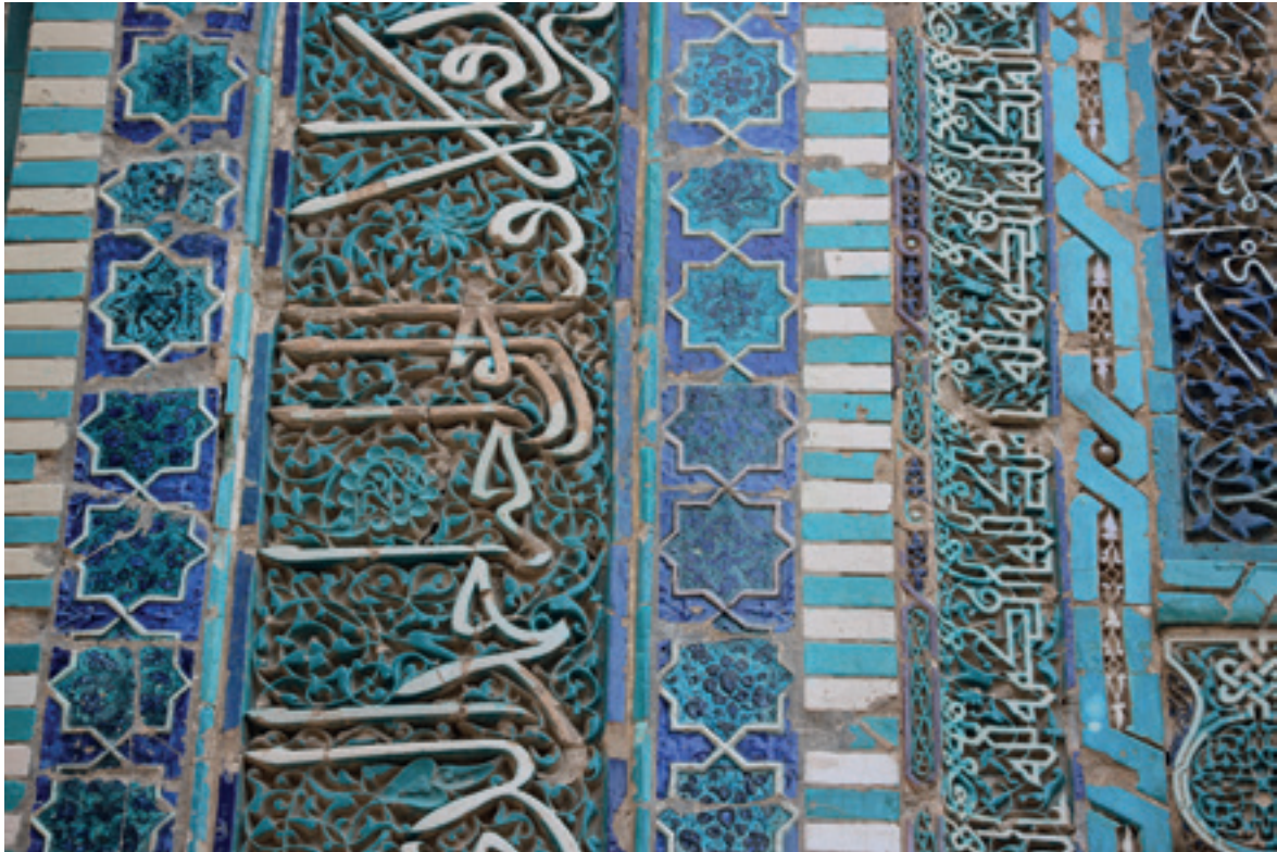
Figure 2. Hodja Ahmad Mausoleum, Framing bands of the façade
